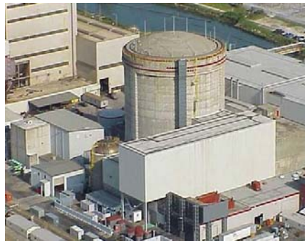
Crystal River Unit 3 Nuclear Power Plant
