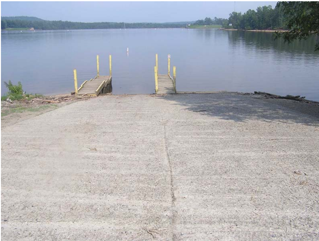
Figure E8-15 View looking south toward Blewett Falls Dam from Pee Dee public access with water surface approximately 2 ft below normal maximum elevation at Blewett Falls Dam.
