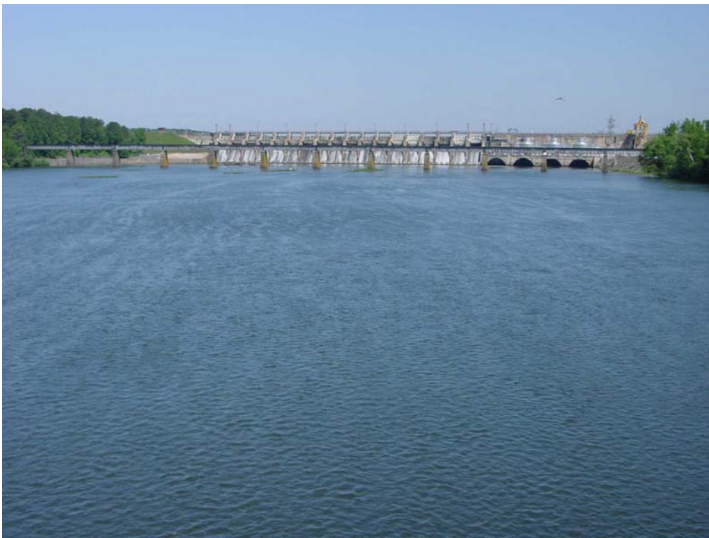
Figure E8-8 View looking upstream towards Tillery Hydroelectric Plant from the N.C. Highway 731 Bridge.
