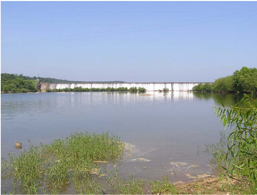
Figure E8-11 View looking north or upstream at Blewett Falls Dam.
