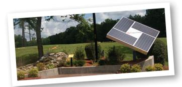
A view of the solar-powered waterfall (on the left) at the entrance to the Harris E&E Center powered by four 170-watt photovoltaic panels. This is equivalent to powering 34 20-watt compact fluorescent light bulbs.
